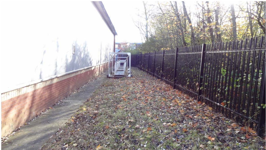
Photo 5: West Elevation viewed from the North
