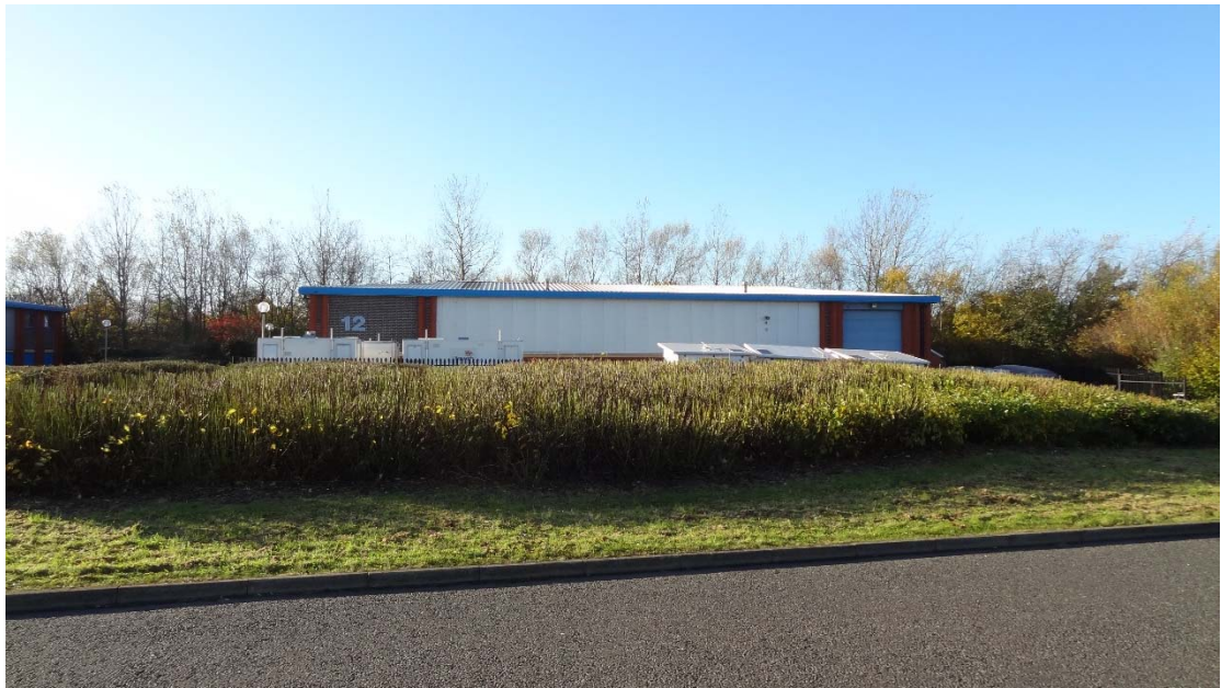
Photo 2: East Elevation viewed from the South
